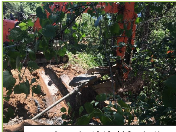
Removing LS 16 old Gravity Line
