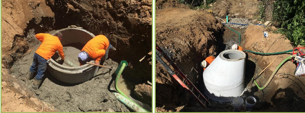
Installing new pour in place Manhole
