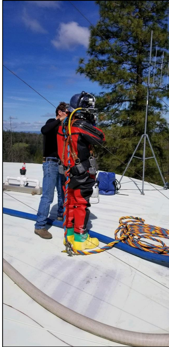
Potable diver gearing up to clean Tank #1
