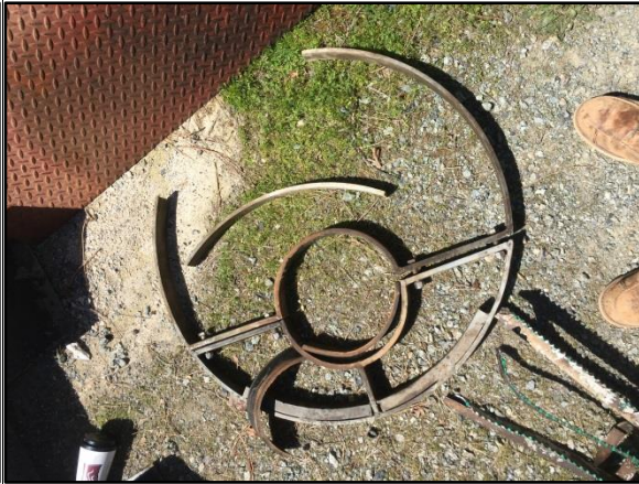
"Centering Spider Rings" had to be cut to finish removal of turbine pump
