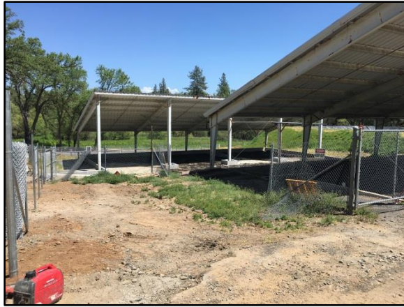
Old fencing that was removed
