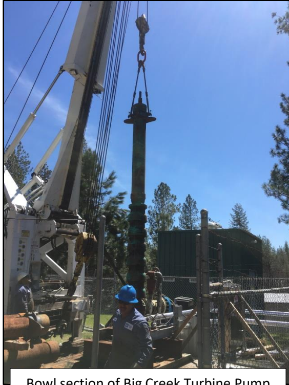
Bowl section of Big Creek Turbine Pump
