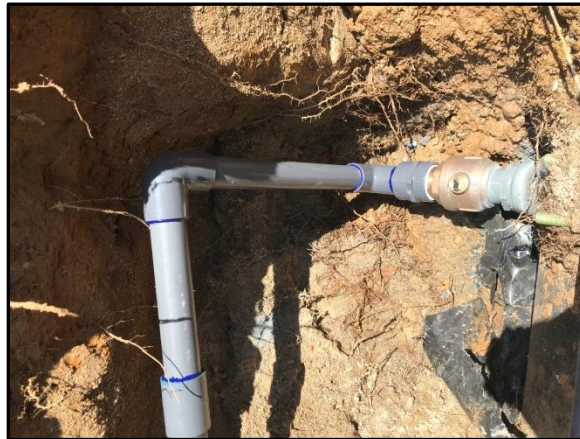
New corporation stop and fittings
