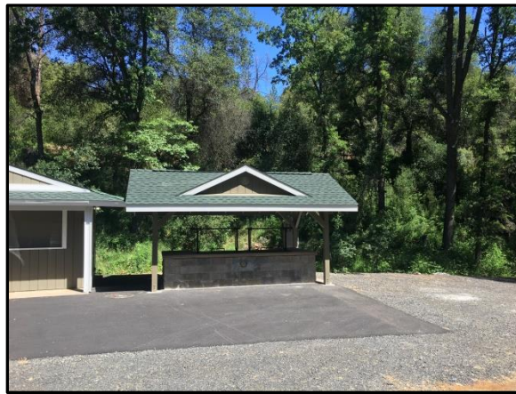
Completed new BBQ pit cover
