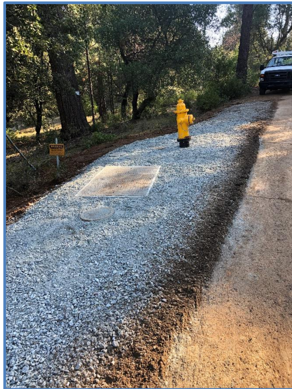
Beck Road High pressure and low-pressure line repair.
