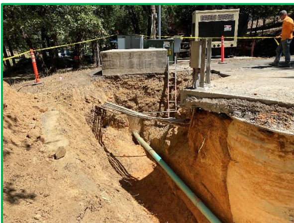
Excavating around Electrical conduits
