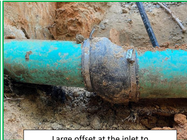
Large offset at the inlet to Lift Station 5
