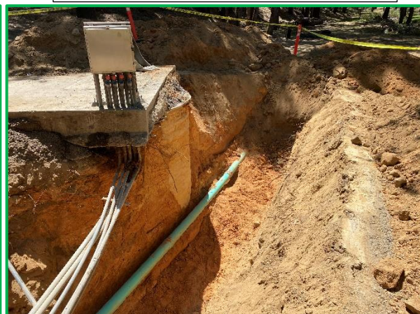
Large offset at the inlet to Lift Station 5
