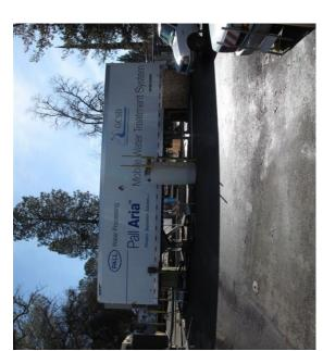
The Pall Trailer is known as the Alternative Water Supply (AWS) treatment plant. The AWS was installed in 2008. It is capable of producing 600 gallons per minute of treated water drawn from Pine Mountain Lake. During a tunnel outage, or emergency situation, the AWS treatment plant is capable of providing a safe drinking water supply to all GCSD customers.
