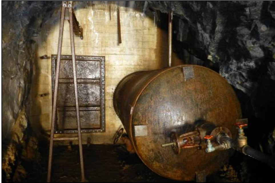
Figure 10: Early Intake adit bulkhead. Capped pipe at right conveyed auxiliary water from the tail race of Early Intake Powerhouse into Mountain Tunnel beginning in 1933. The pipe was capped in 1997.
