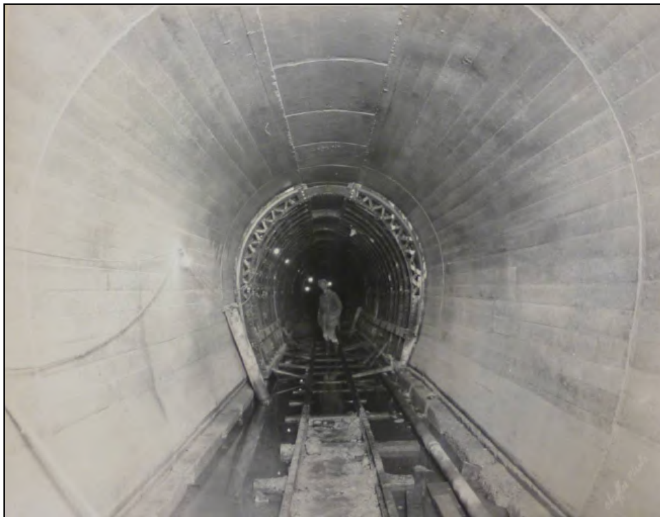
Figure 7: Concrete lined segment of tunnel at Adit 8-9. March 1923.
