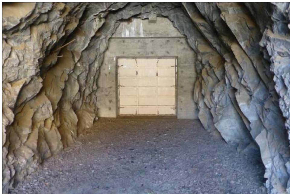
Figure 15: Early Intake Adit. Concrete bulkhead and watertight door installed in 1997. September 24, 2014.
