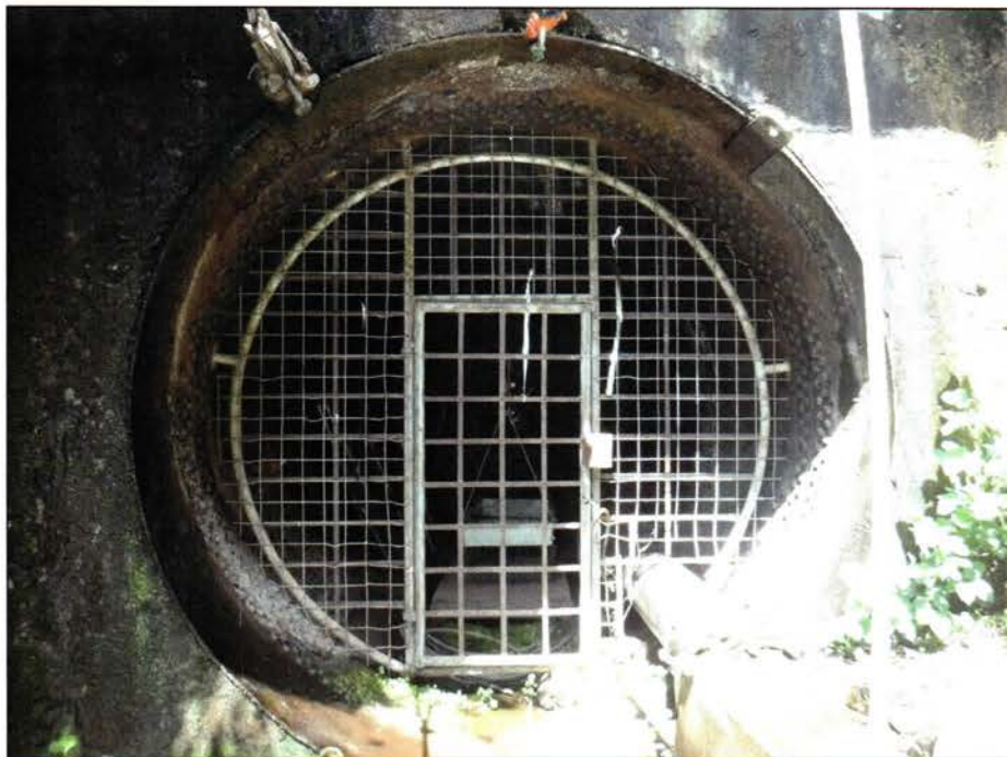
Photograph 3: Detail of South Fork Adit north portal on north side of river with circa 1969 bulkhead door installed after pipeline removal, view facing north, May 3, 2018 (AECOM).
