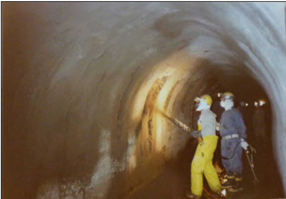
Photograph 13: Crews lining Mountain Tunnel at the South Fork crossing in 1990. 3
