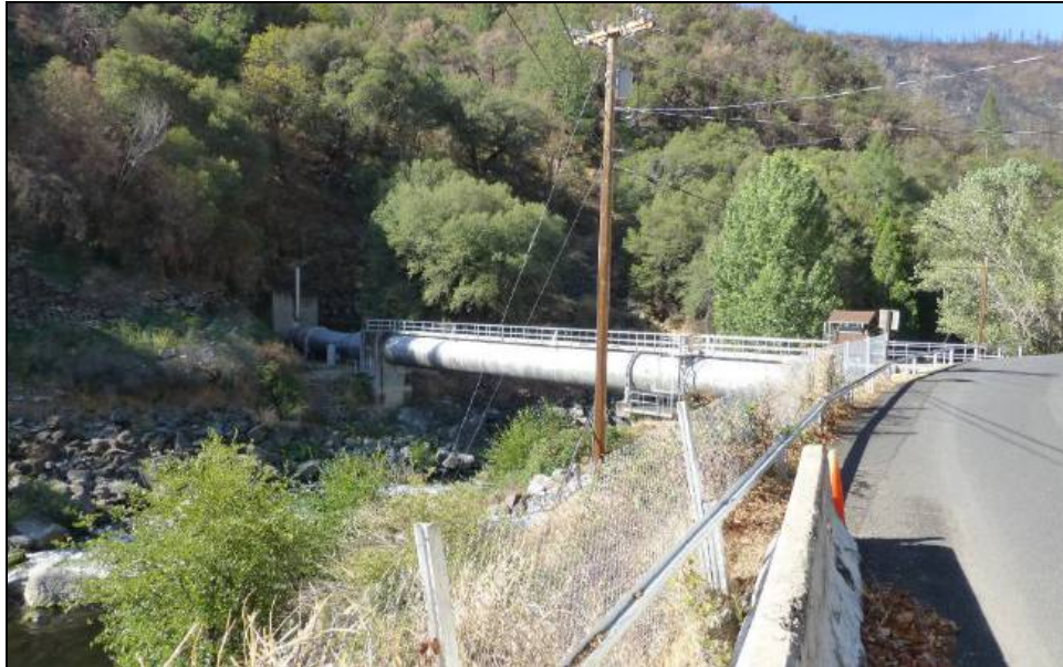
Figure 12: Bypass tunnel across the Tuolumne River is one segment of a bypass tunnel constructed in the mid-1960s to convey water from the Kirkwood Powerhouse tail race into Mountain Tunnel. This is currently the functional intake to Mountain Tunnel. September 24, 2014.
