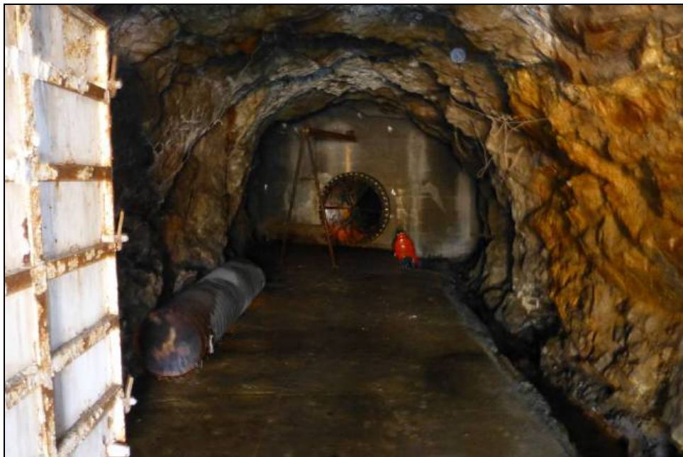
Photograph 23: Adit 5-6 (MT-5), showing open watertight door at left and concrete seal with 60-inch watertight cover, and an orange valve weeper. Note the drainage channel at right. Camera facing south, September 24, 2014.
