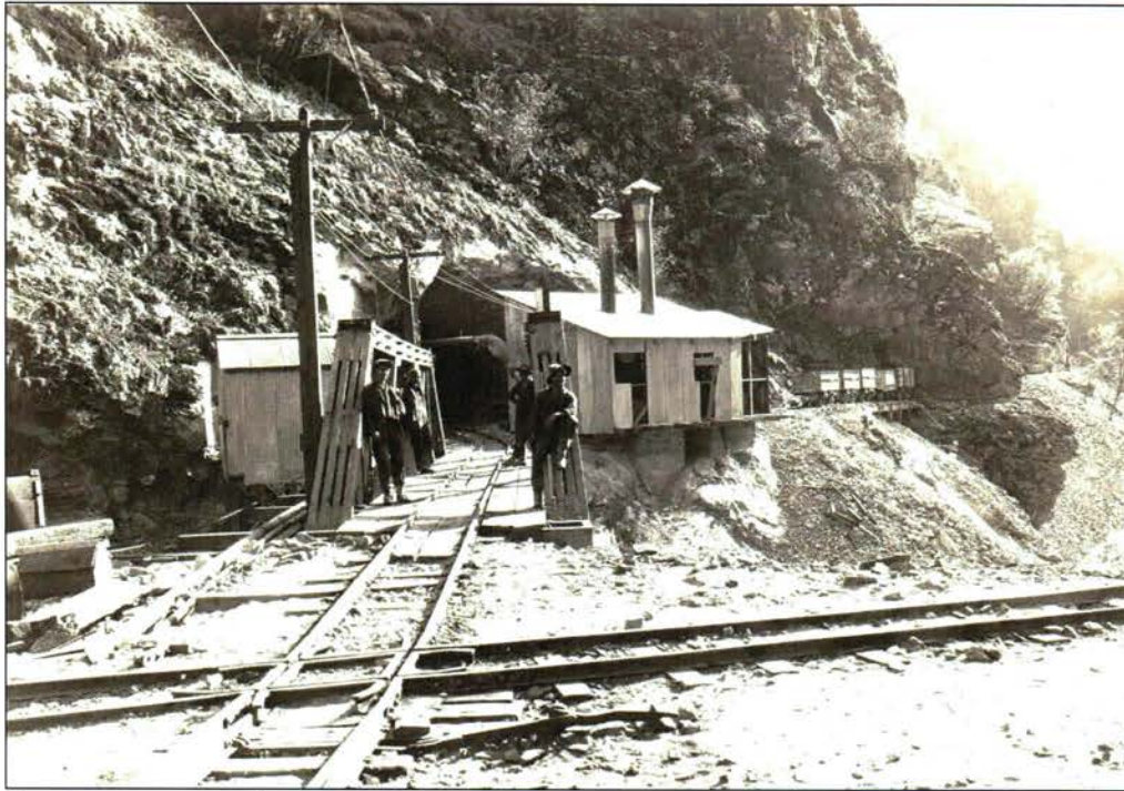
Plate 2: August 1921 photograph showing South Fork Adit on south side of river, temporary bridge, and camp buildings prior to construction of the piped section of the Mountain Tunnel (c. 1921-1924). (Courtesy of Hetch Hetchy Water and Power Records and Archives, HHWP #246306.)
