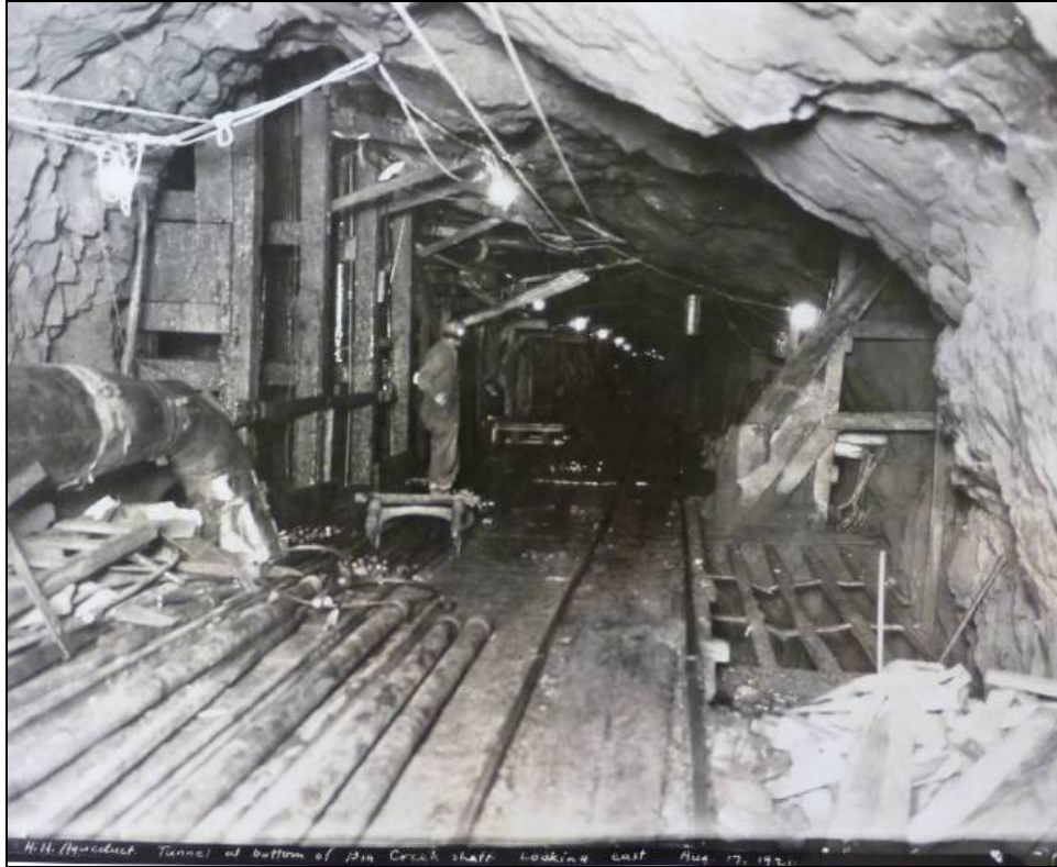
Photograph 30: 1921 photograph showing the junction of Big Creek Shaft (MT-7) with Mountain Tunnel. Photograph courtesy of Moccasin Archives.
