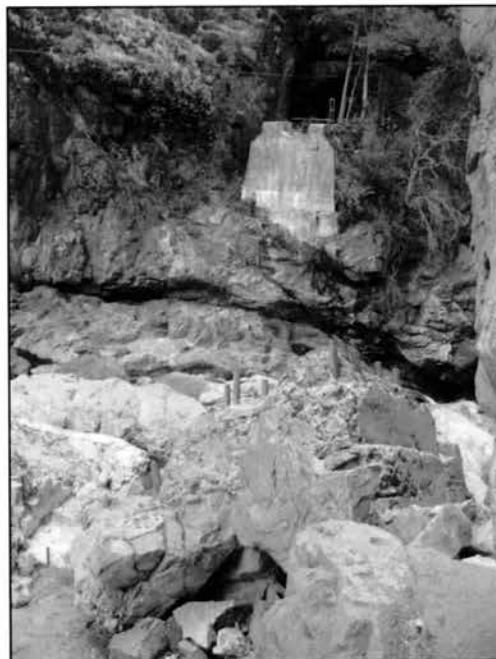
Photograph 4. View southwest showing collapsed support pier.
