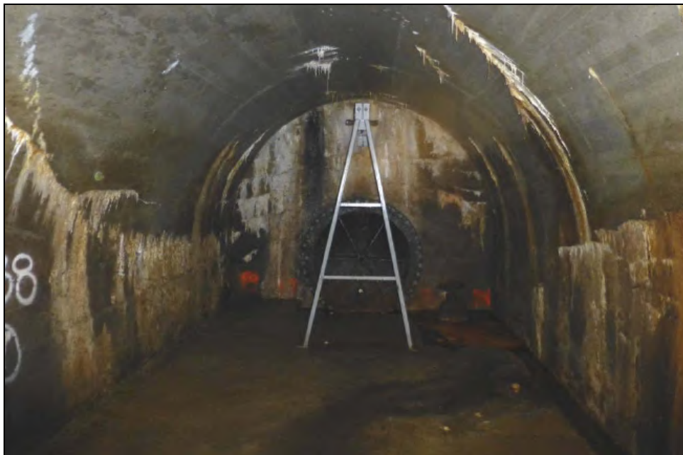
Photograph 27: Adit 8-9 (MT-6) looking towards concrete seal with 60-inch watertight cover, and an orange valve weeper. Note the drainage channel at right. Camera facing south, September 24, 2014.
