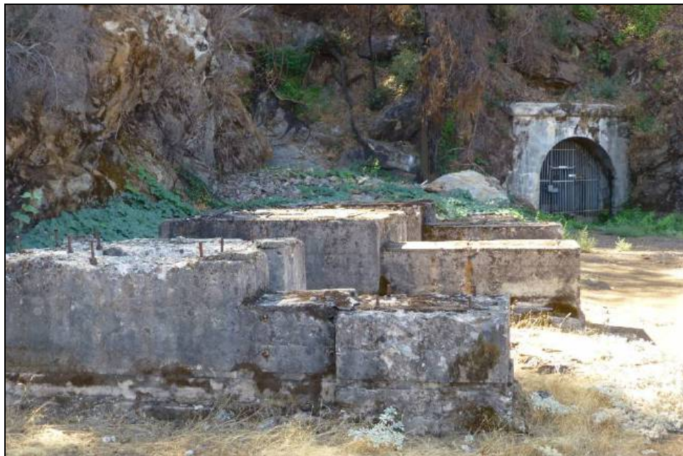
Figure 3: Foundations for compressors shown in Figure 2 remain outside of Adit 5-6. September 25, 2014.
