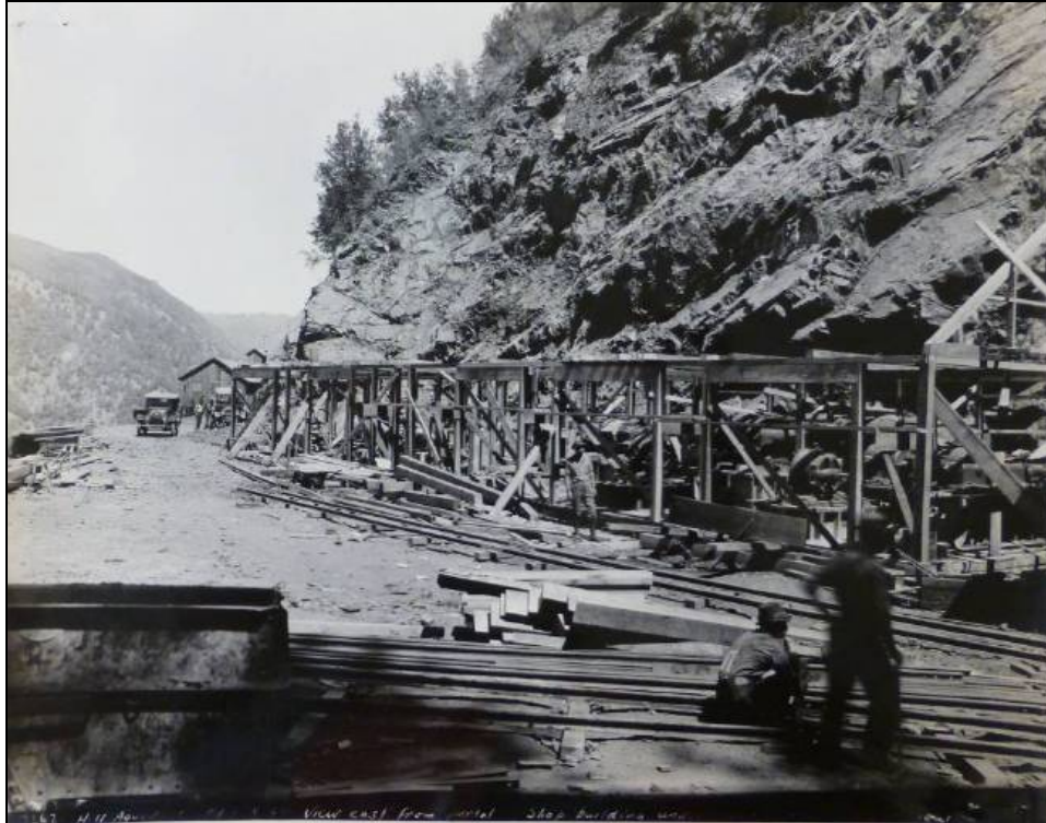
Photograph 24: Historic photograph, circa 1920, showing construction of compressor house outside Adit 8-9 (MT-6). Photograph courtesy of Moccasin Archives.
