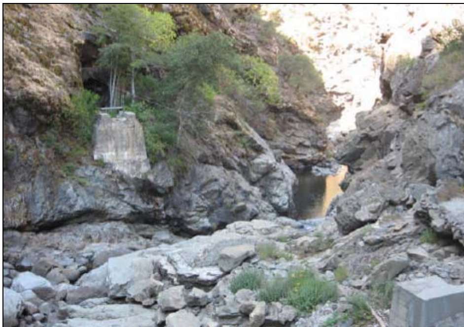
Figure 13: South Fork crossing in 2008. Note remnant concrete piers at bottom right and left that supported the original pipeline crossing the river. Photo credit William Self Associates, Inc. 35
