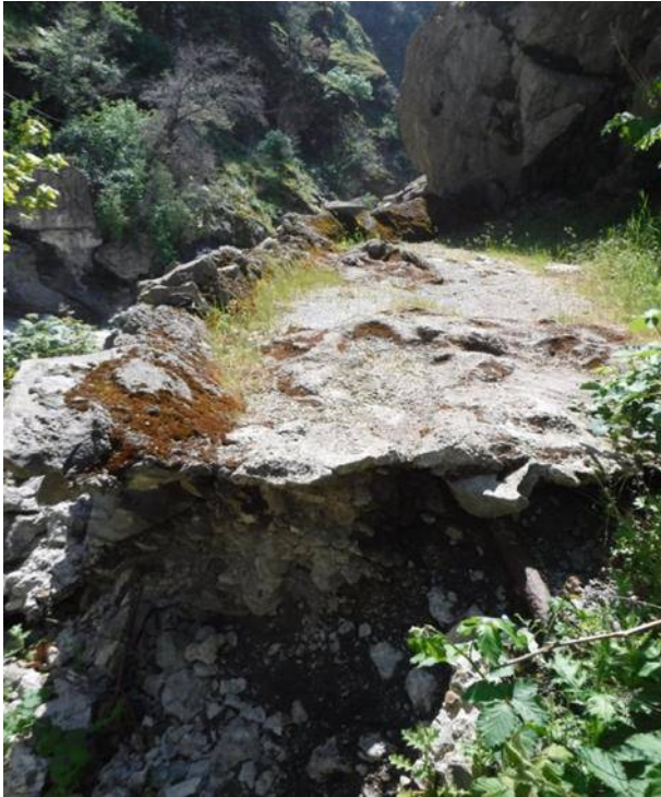
Photograph 2: Shotcrete surface and rubble base. View southwest. Field-designated Context 2.
