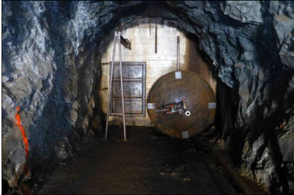
Photograph 18: Early Intake Adit (MT-2) concrete seal with manhole and capped pipe connection from Early Intake Powerhouse tailrace. Camera facing south, September 24, 2014.
