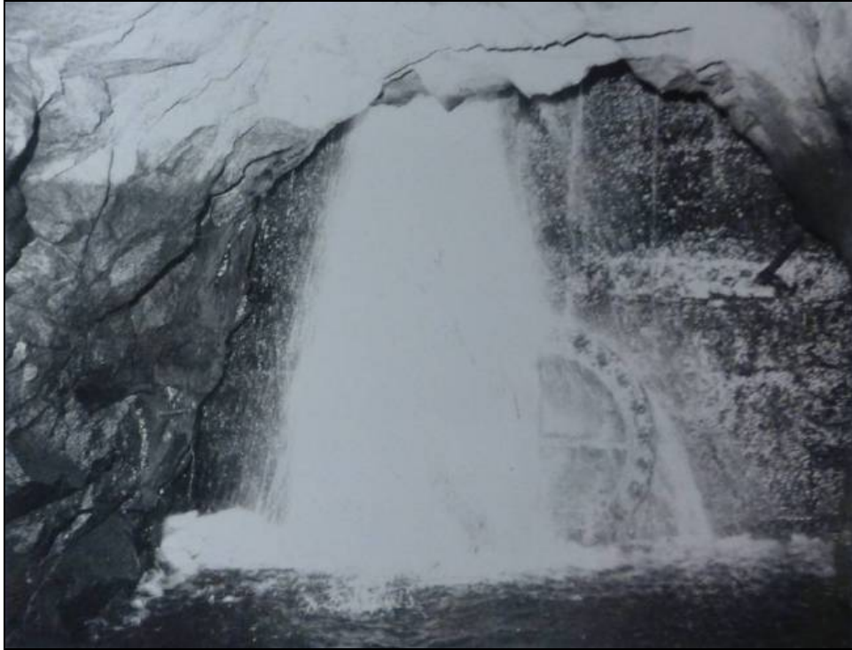
Photograph 20: 1972 photograph of Adit 3-4 (MT-3) showing water breach. Photograph courtesy of Moccasin Archives.
