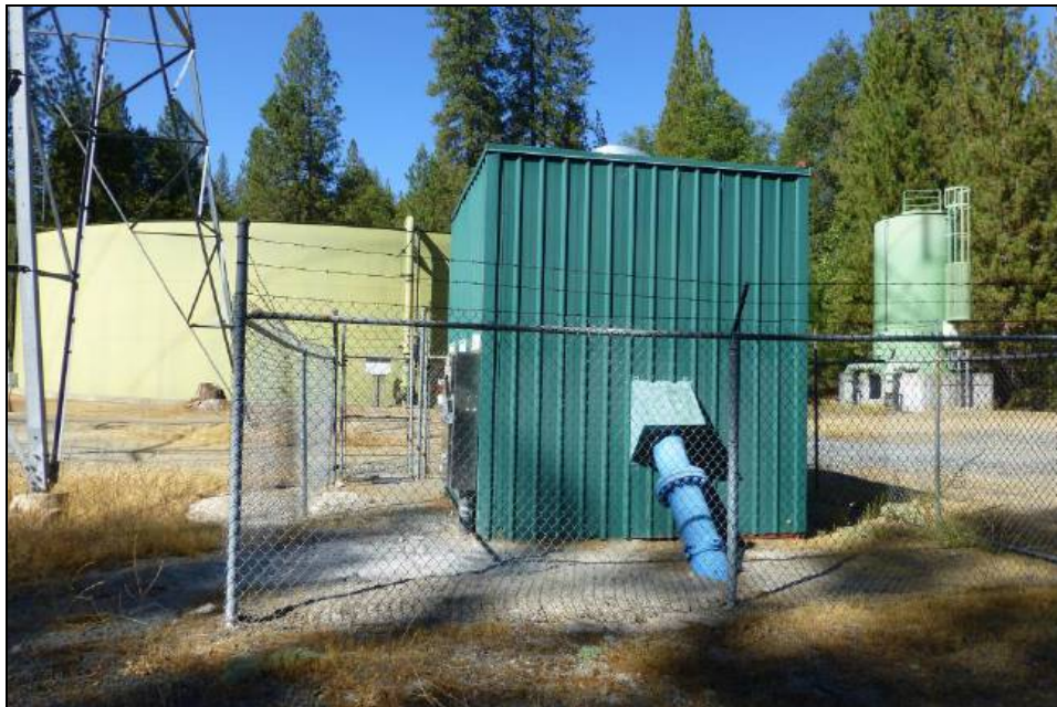
Photograph 29: Big Creek Shaft (MT-7) pumphouse. This shaft, used to access driving faces during construction of Mountain Tunnel now supplies water to a local district. Camera facing north, September 24, 2014.
