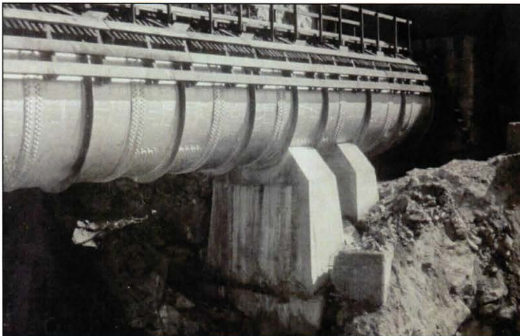
Plate 3: May 1925 photograph of riveted pipe segment of the Mountain Tunnel entering south portal adit and concrete piers on south side of river. It is unclear if both piers are still extant. (From JRP's 2015 Mountain Tunnel DPR 523 form.)
