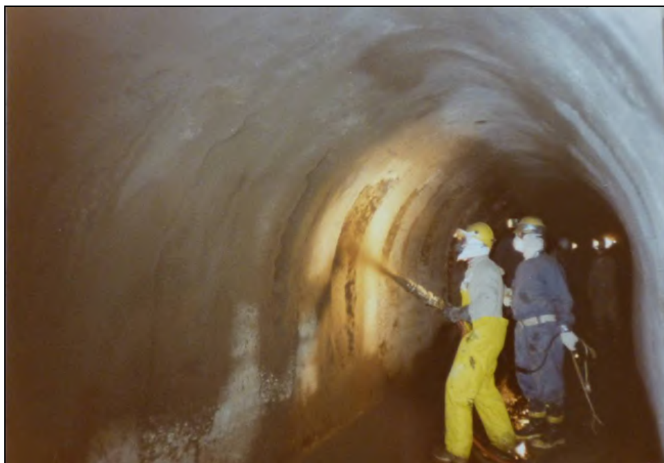
Figure 14: Crews re-lining Mountain Tunnel's siphon at the South Fork crossing in 1990.
