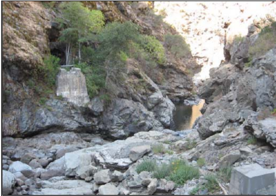
Photograph 12: South Fork crossing in 2008. Note remnant concrete piers at bottom right and left that supported the original pipeline crossing the river. Photo credit William Self Associates, Inc. 2
