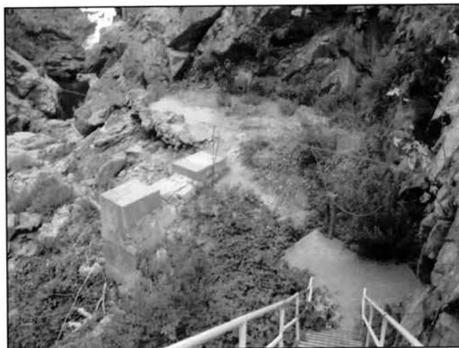
Photograph 6. View west from access road showing shotcrete reinforcement (above pier), and access cable.
