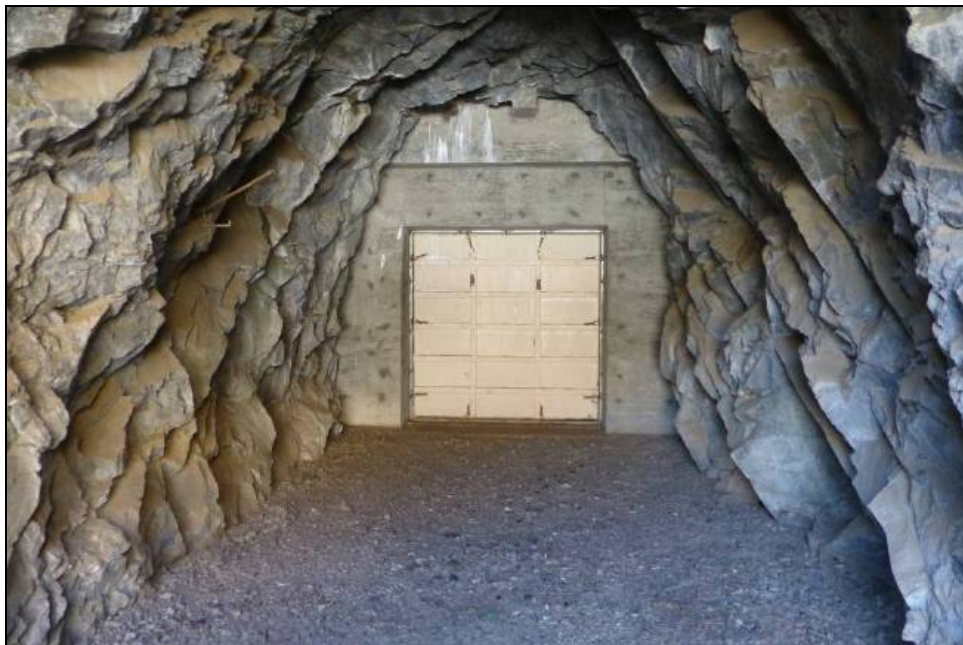
Photograph 17: Early Intake Adit (MT-2), concrete bulkhead and watertight door installed in 1997. Camera facing south, September 24, 2014.
