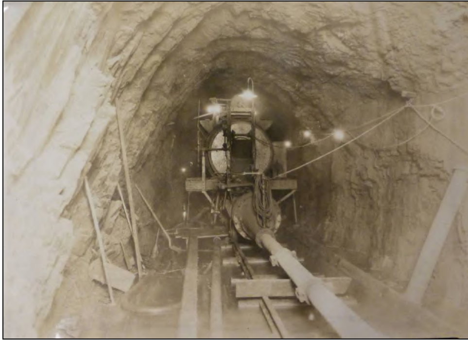
Figure 6: Concrete gun applying lining to tunnel at Adit 8-9. March 1923.
